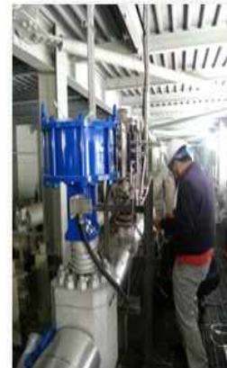
ANSI Class 4,500 pressure control valve at Yeongheung thermal power plant in Korea
